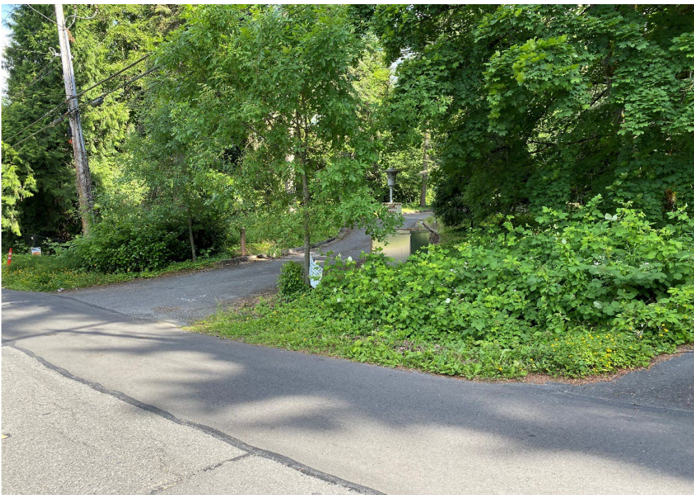
View of existing paved access drive to pump station.
